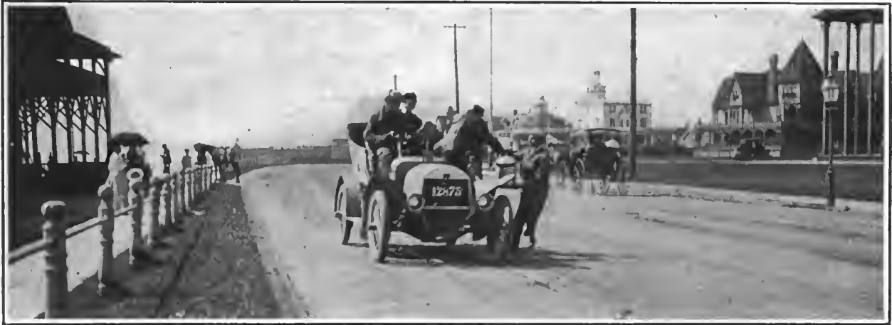
PASSING FUEL SUPPLIES TO THE FRAYER-MILLER AIR-COOLED CAR IN THE NONSTOP-ECONOMY TRIALS AT LONG BRANCH, NEW JERSEY—THIS CAR WON THE CONTEST, COVERING 2,915 MILES IN 143 HOURS, 46 MINUTES.
